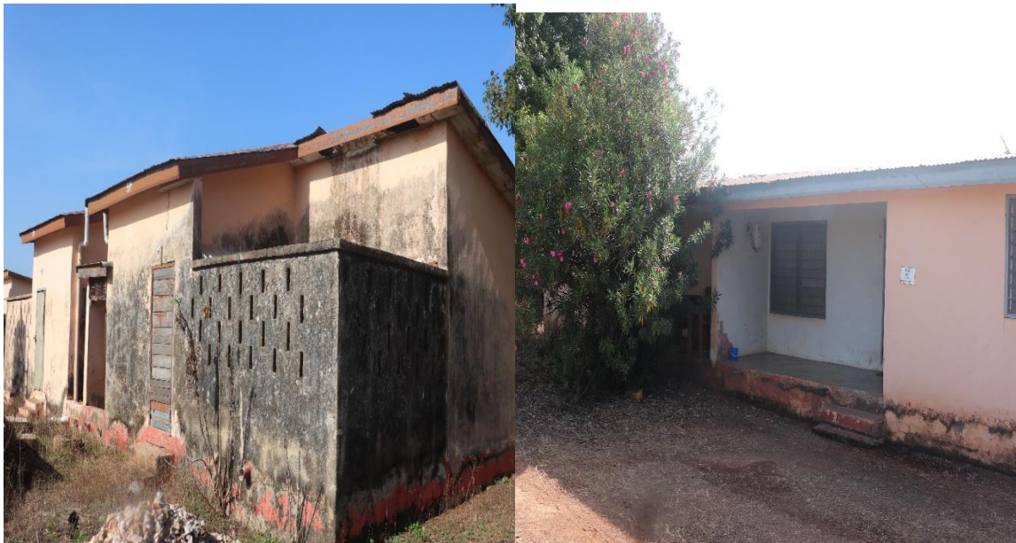
Photos of back and front view of the Bolga building
