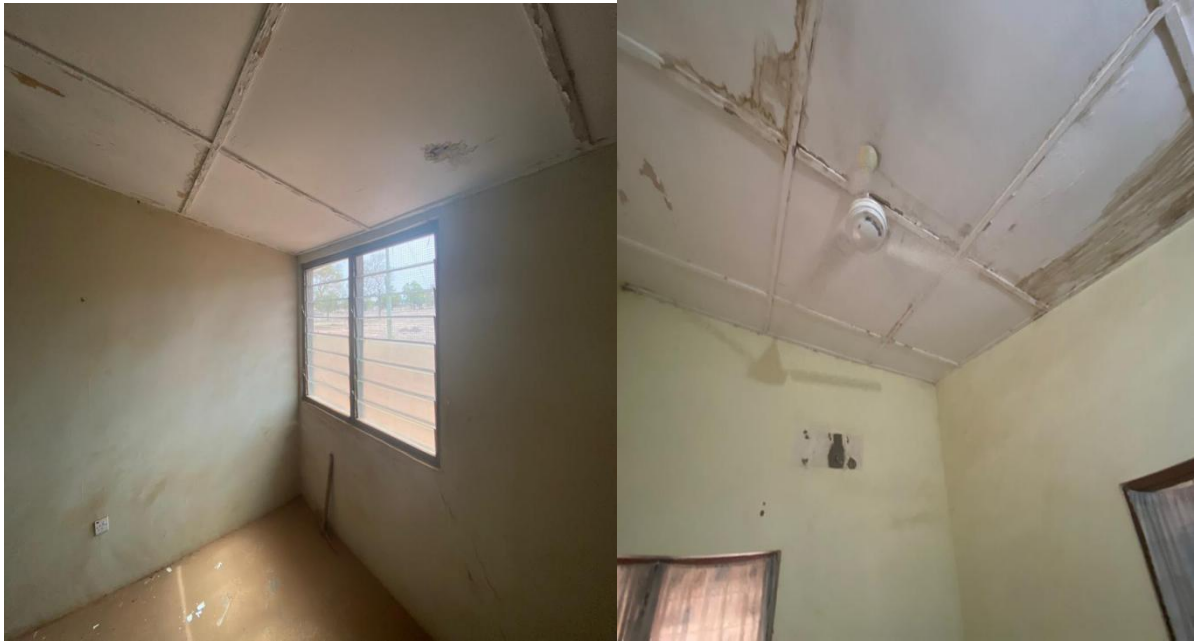
Ceiling, walls and floor of the building
